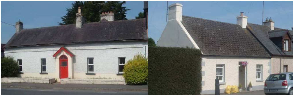
Vernacular farm cottage with Arts and Crafts style porch, one-over-one-sash windows, replaced with uPVC (left). This small, quaint cottage is one of a group, although this is the one with the fewest alterations, and is indicative of what much of the village would have looked like in the nineteenth century. The roof would have originally been thatched. Note the sliding timber windows (right).
