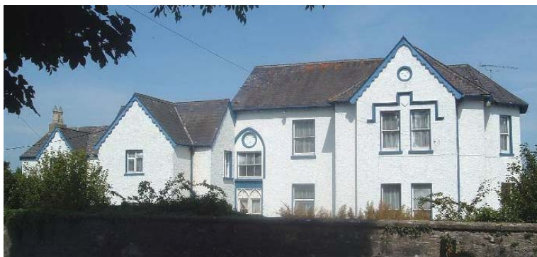
Nursing home, dating from the late nineteenth century, once Lisbrack House and home to Bishop Conroy. Note the Dutch influence in the triangular Arts and Crafts gables, the bay windows and the timber bargeboards.
