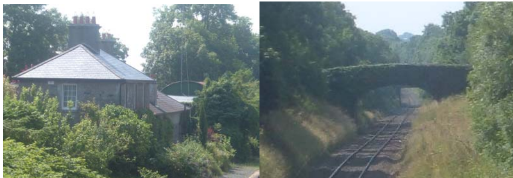
The Station, which was built at the time of extensive railway construction during the 1860s, was closed in 1963 and is now a residence. This is an attractive ashlar limestone building, with a hipped slate roof. The station building once housed the station ticket office, waiting rooms etc on the ground floor and living accommodation for the stationmaster and his family on the first floor.
