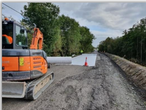
Restoration improvement works on the R398 in Ballymahon MD
