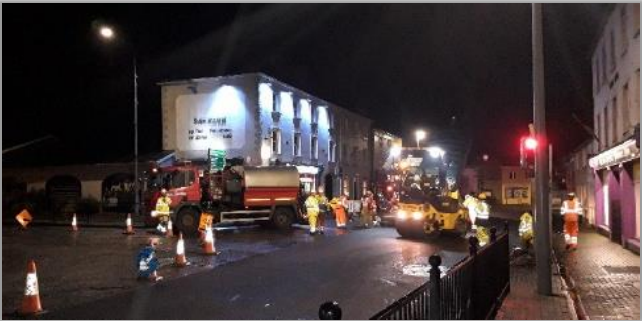
Night-time Pavement Works in Edgeworthstown
