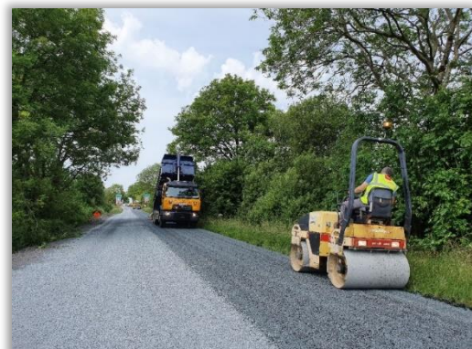
Surface Dressing Works on the N63 at Barnacor in Ballymahon MD
