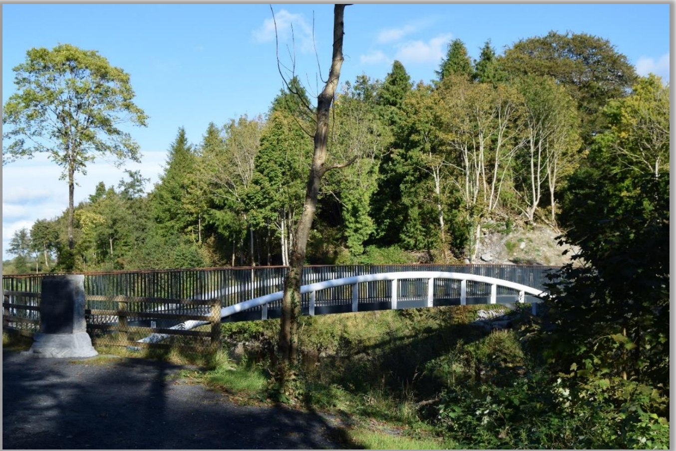
The White Bridge at Newcastle Woods Walking Trail
