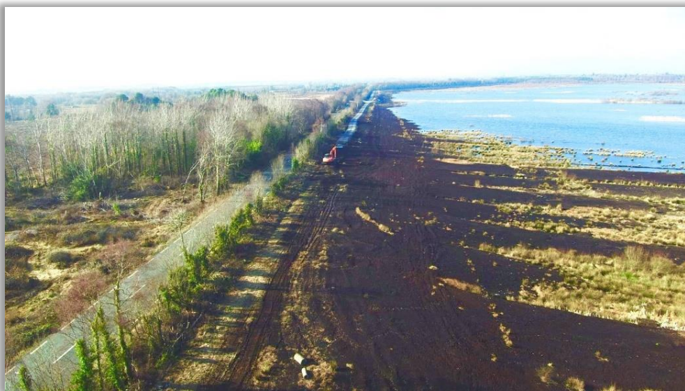
Corlea Amenity Walk Phase 2 pictured during construction
