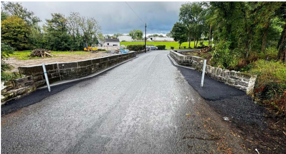
Kilnacarrow Bridge, Ballinalee
