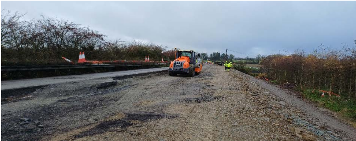
N55 Royal Canal Way – Emergency works
